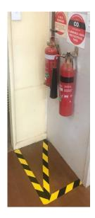
The exclusion zone markings are in several locations to ensure that no items of any kind are placed on the floor that might obstruct access to the fire extinguishers or to the electrical panel.
